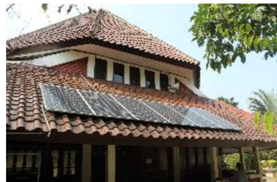
Solar Panel Mushola FIB
