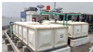
Gambar 6.7 IPAL di IMERI Figure 6.7 STP at IMERI
