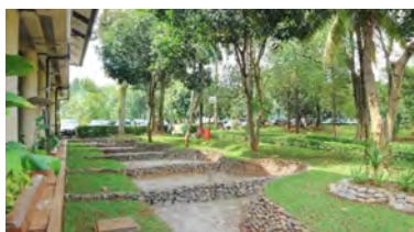
Gambar 6.6 Sistem Panen Air Hujan di Fakultas Teknik Figure 6.6 Rain Water Harvesting at the Faculty of Engineering
