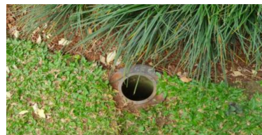
Gambar 6.9 Lubang Resapan Biopori Figure 6.9 Biopore Infiltration Hole
