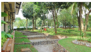
Gambar 6.6 Sistem Panen Air Hujan di Fakultas Teknik Figure 6.6 Rain Water Harvesting at the Faculty of Engineering
